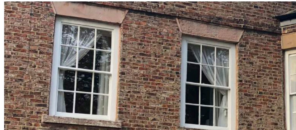
ORIGINAL SASH WINDOWS
